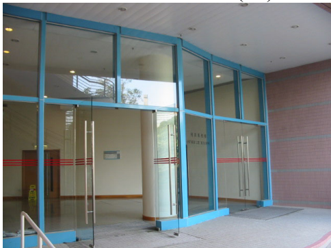
ELB main entrance (P5)
